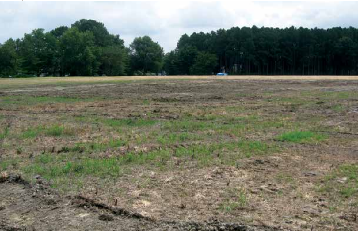
This photograph shows the wetland immediately post-restoration before it filled with rainwater.
